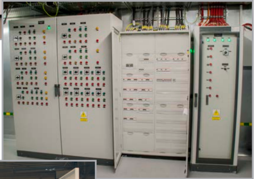
Ventilation systems control panel, line II of Warsaw Metro
