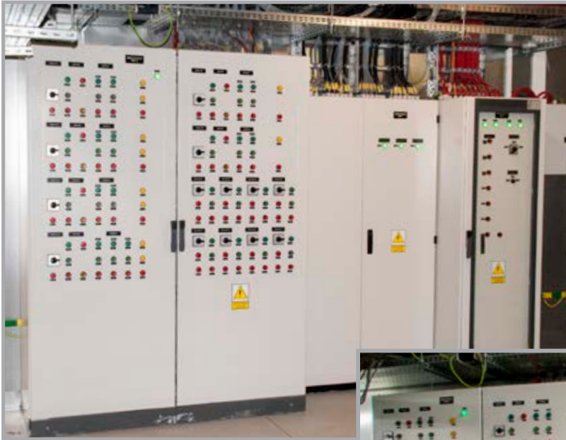
Ventilation systems control panel, line II of Warsaw Metro
