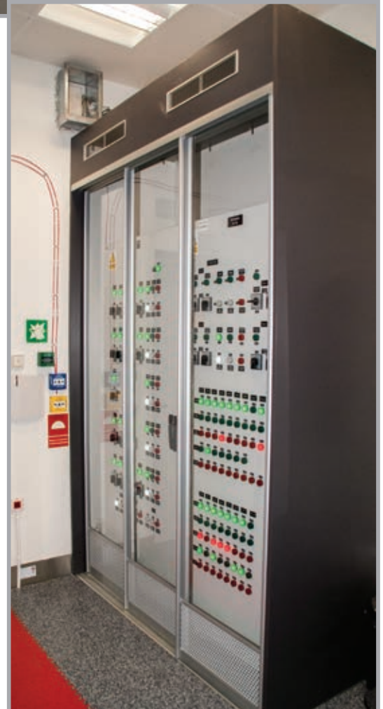
Electrical lighting control panel, line II of Warsaw Metro
