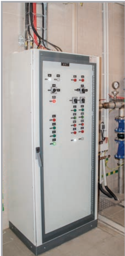
Pumps control panel, line II of Warsaw Metro
